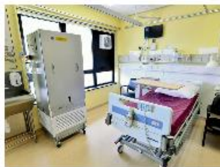
Provision of HEPA filter next to the window
